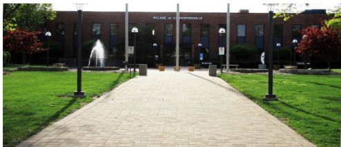
Carpentersville Branch Court
